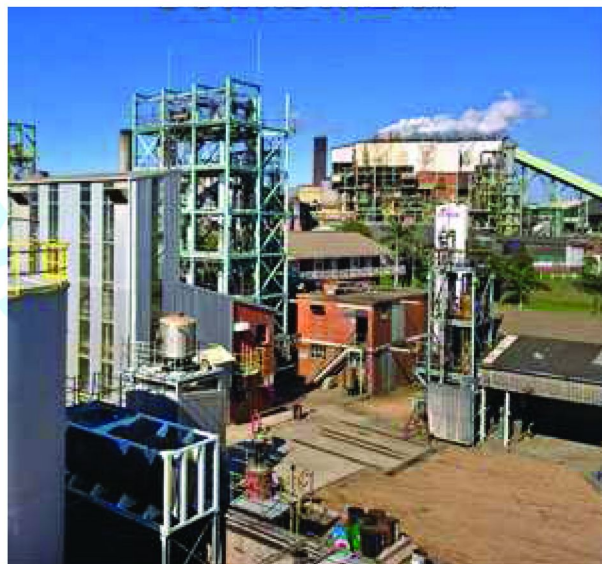
Figure 3. The Sezela furfural plant on the south coast of KwaZulu-Natal in South Africa
